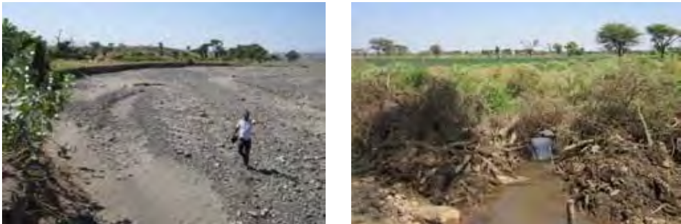
Figure 6: Left: Bank erosion encroachment of agricultural land; Right: Onion irrigated from Kebena river regard to embankment protection, localized bed stabilization as well as construction of intakes and canals with the objective of making better use of the hugely underutilized Kebena river flow (figures 7 and 8).
