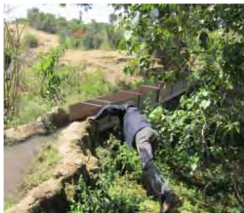
Figure 26: : Flume on branching canal to cross a gorge
