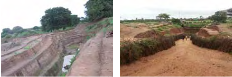
Figure 32: Left: Unprotected embankment of livestock corridor and Right: Protected embankment of livestock corridor.
