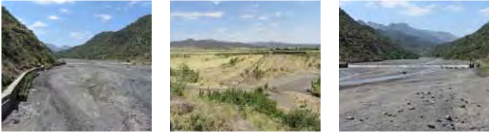
Figure 36: View of the Alewuha scheme
