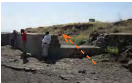
Figure 13: Opening made for intake on the wing-wall of the Hara spate irrigation scheme
