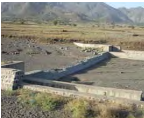
Figure 12: Headwork, diversion structures of the Hara spate irrigation scheme
