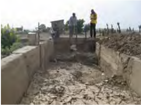
Figure 29: Sediment in the canal of the Bura system
