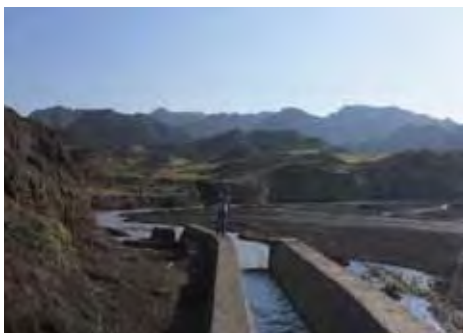
Figure 34: The Andina Mellie headwork structure
