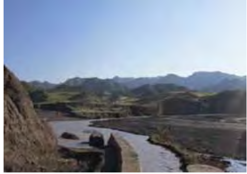
Figure 35: Main canal breached (left) and open off take structure showing the toppled retaining wall
