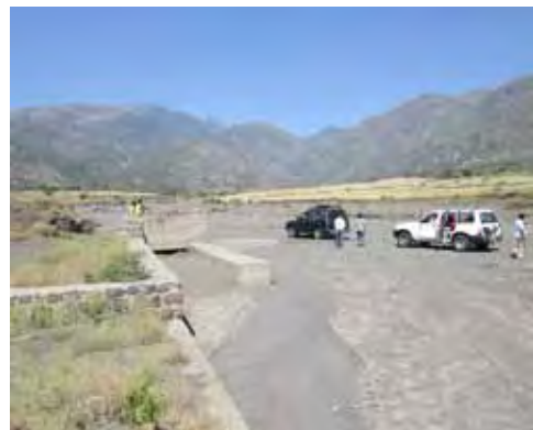
Figure 12: Headwork, diversion structures of the Hara spate irrigation scheme
